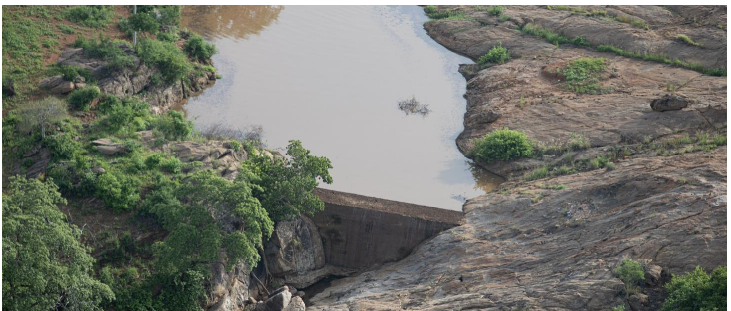
The photo above shows Rhino Valley Sand Dam filled with water following the March and April rainfall, reflecting the strong seasonal recharge across the landscape. The recent rains have also contributed to increased sand accumulation in various sand dams, accelerating their maturation and improving their long-term water storage capacity. Photo Credit: Tsavo Trust – Joseph Kyalo.
