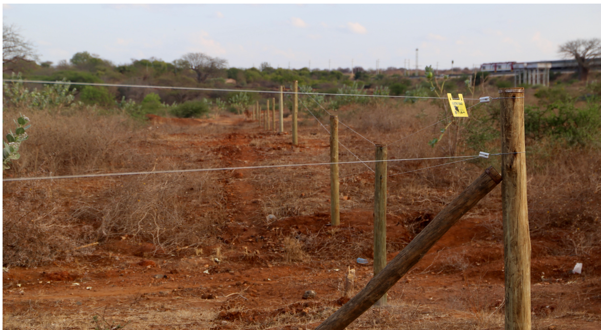
Below: Photo shows the 2 strands of wire, 5 foot off the ground (allowing passage of livestock underneath) and the 3 rd wire is the earth, set underground. This fence configuration is a tried and tested HEC mitigation system that has worked well.
