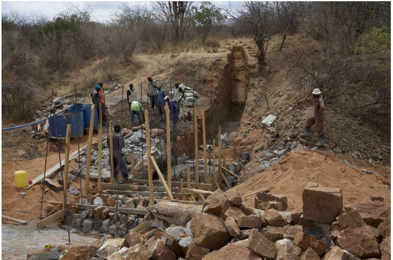
Kangechwa B sand dam under construction and expected to be completed by mid-November 2020 in anticipation of the rainy season. Sand dams are a tried and tested water catchment method in arid lands and have proven to be environmentally friendly and very effective with little desertification around the water catchment. This is in contrast to the bore hole system that has proven over and over again, in many Protected Areas, to cause great environmental vegetation desertification around the eye of the bore hole water supply.
