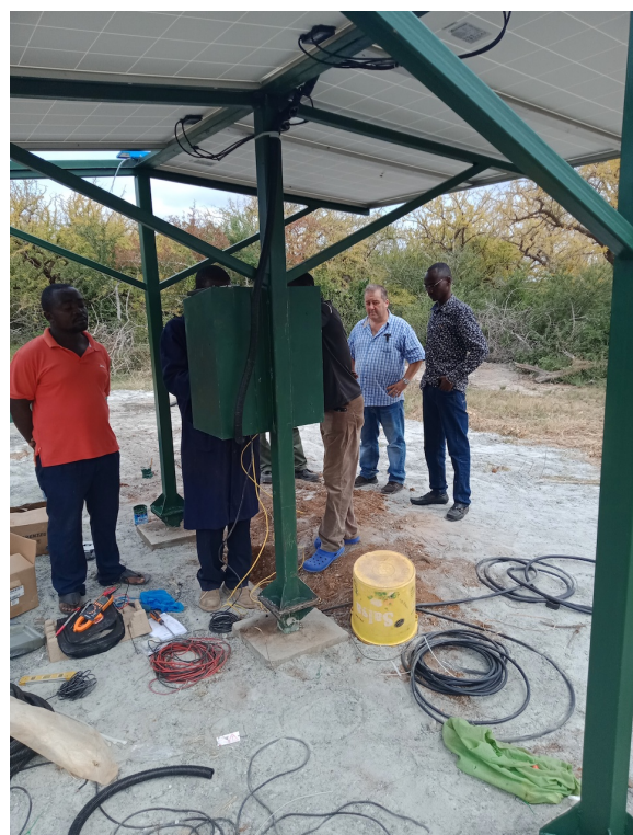
Right: Training meeting at Shirango borehole site where solar panels have been installed to pump water, Jan20
