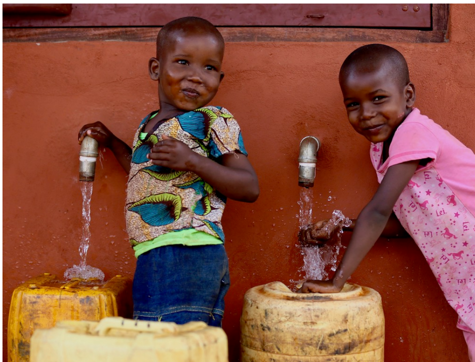
Photo shows 2 happy Kamungi kiddies enjoying water on tap for the first time on 31 st October 2017 at the water dispensing kiosk at Ngiluni village.
