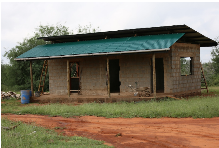
TENP Dakota Base – 1 of 2 three room Ranger blocks in final stages of completion – November 2018
