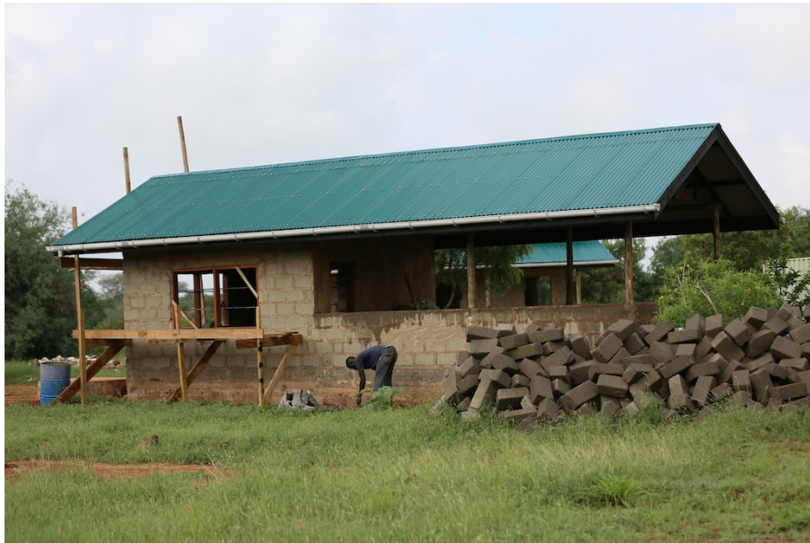
TENP Dakota Base kitchen / Mess building in finishing stages - November 2018
