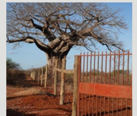
Solar powered electric fence around Dispensary
