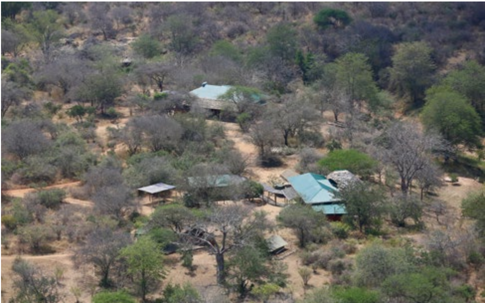
Aerial photo showing the new houses at Tsavo Trust HQ in 2018. Each house has 2 bedrooms, en-suite, kitchen, solar power and water heating and completed to a high standard
