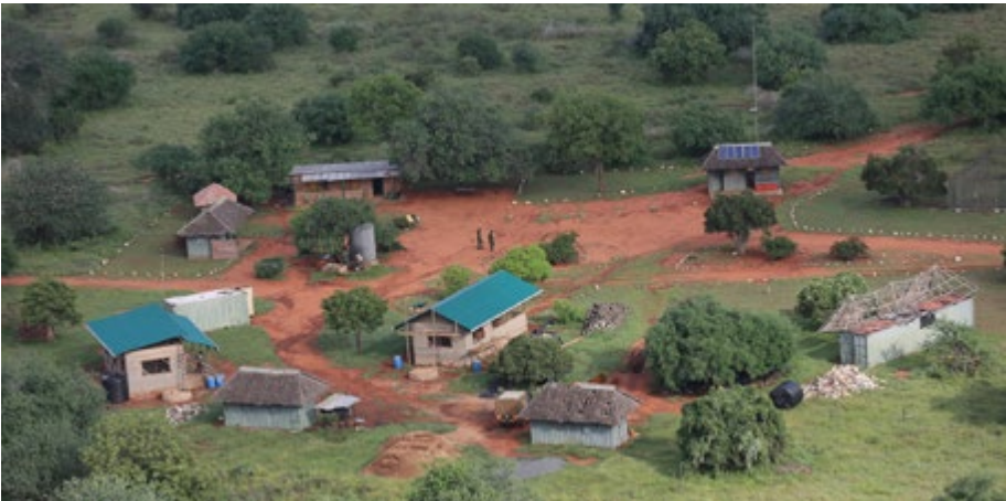
December 2018: KWS Dakota Base upgrade, ranger accommodation and facilities - works in progress.
